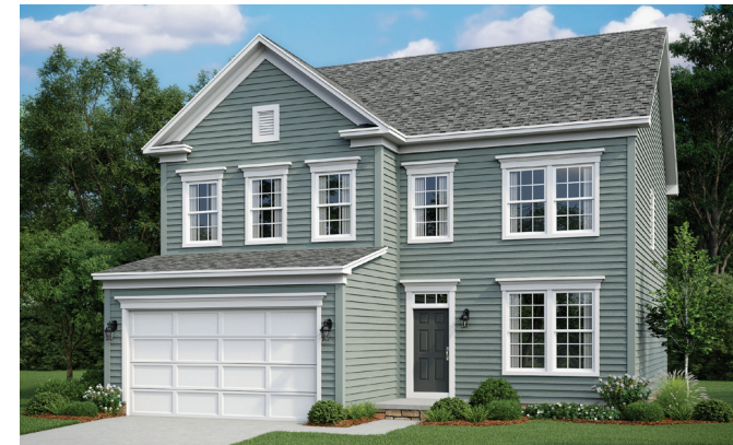
{ Eastern Seaboard Stone to Grade }
